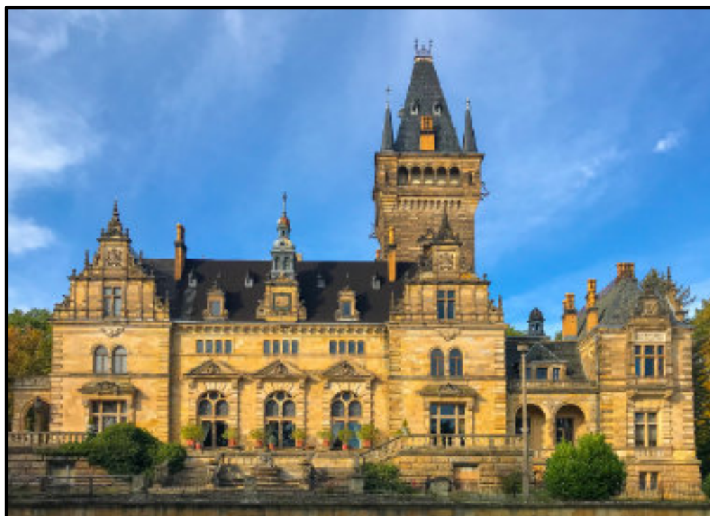
The hunting lodge in Hummelshain was built in the 1880s. It was an impressive structure but appeared to be in a state of disrepair.
